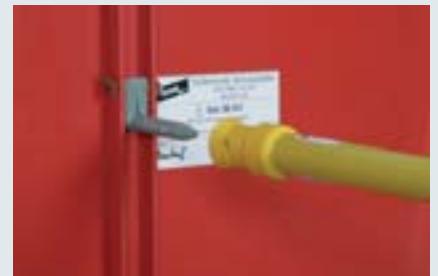
Operating rod with T pin shaft (bayonet) and insulating protective shutter with T pin shaft coupling.
