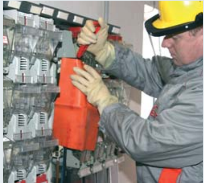
Live working with insulated gloves at voltages up to 1000 V.
