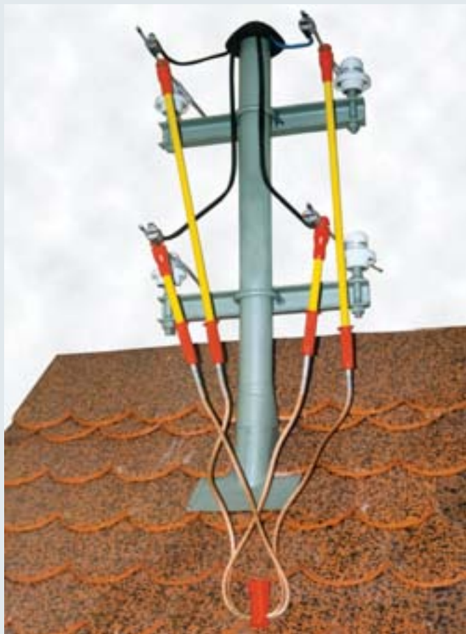
Sample construction of a four-pole short-circuiting device.
