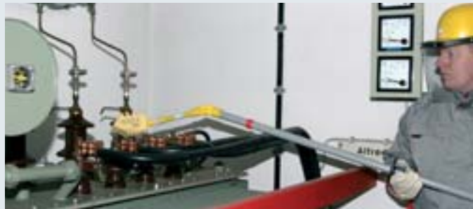
Dry and damp cleaning of a transformer under live conditions with TFRS MS Combined Cleaning Set.
