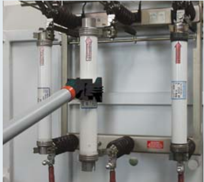
Angled (20°) SZ fuse tongs for installing and removing h.v.h.b.c. fuses.
