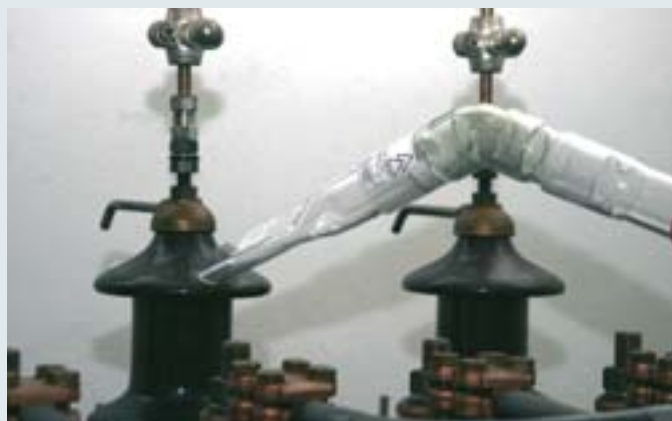
Cleaning an insulator with a flat cleaning head and angled intake tube (135°).
