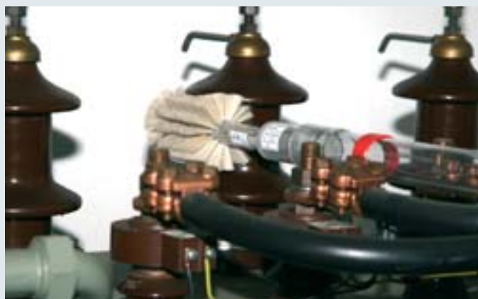
Cleaning an insulator with a tubular brush.
