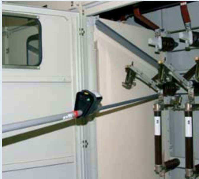
PHE Voltage Detector with visual indication used in a switchgear installation.
