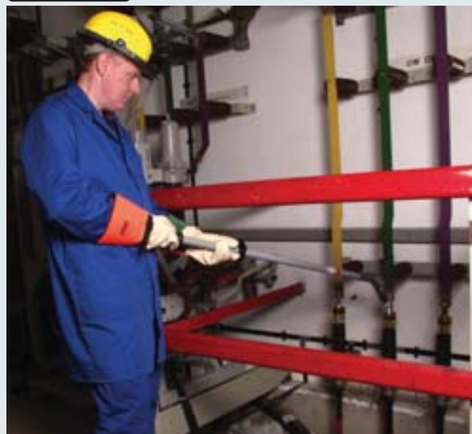
Opening the sealing screw with the MS insulated screw driver.
