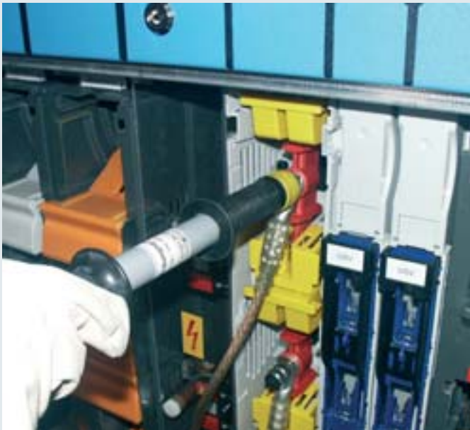
Installing the partly insulated earthing and short-circuiting device with earthing handle Type TI
