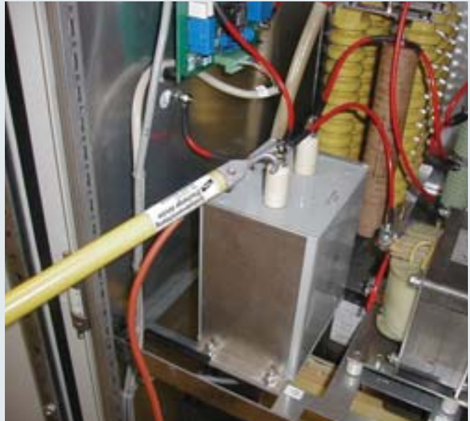
Single-pole device for discharging static charges.
