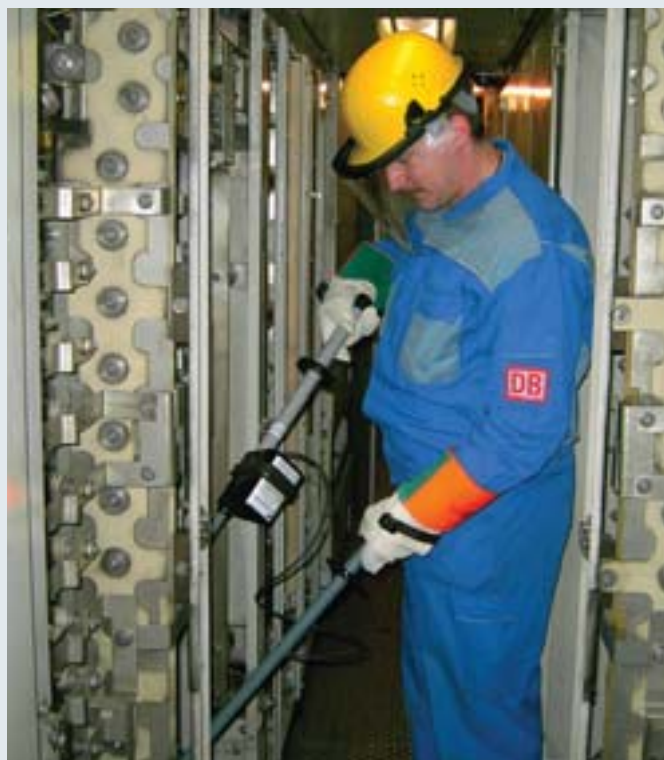
PHE/G II dc voltage detector for intermediate dc circuits (ICE operating head).
