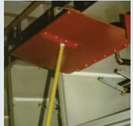
Inserting of an insulating protective shutter, Type A3, by operating rod
