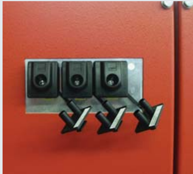
Passive DEHNcap/P voltage detector used for an encapsulated switchgear installations.
