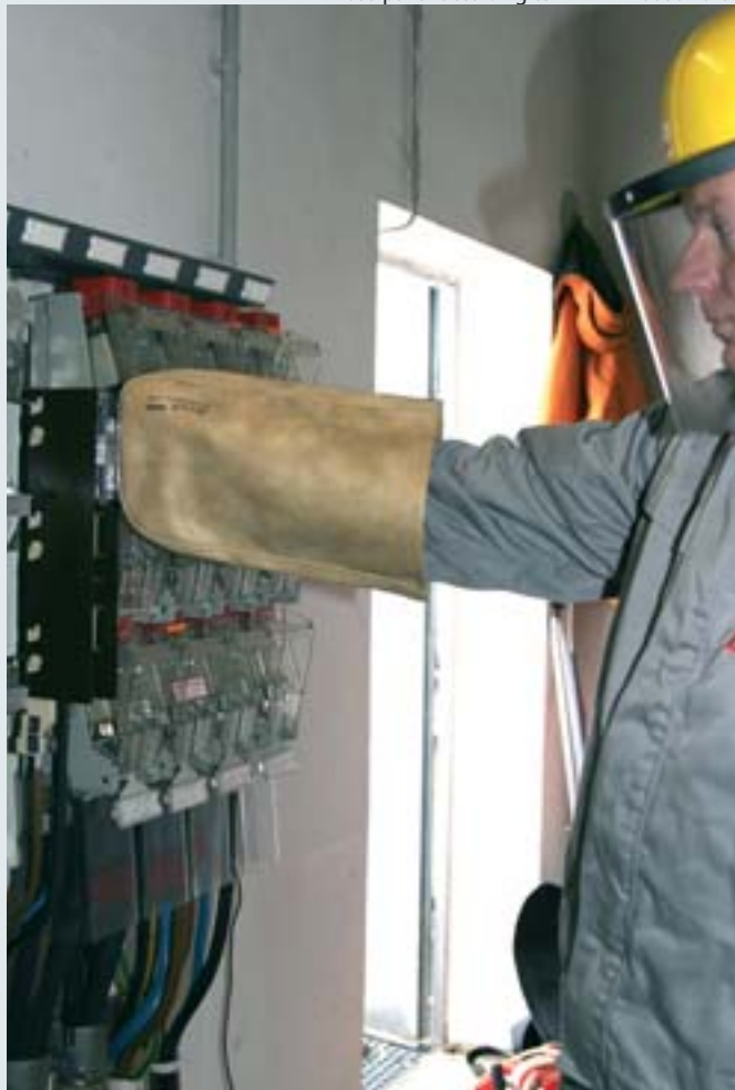
Inserting an NH fuse with the necessary personal protective equipment.
