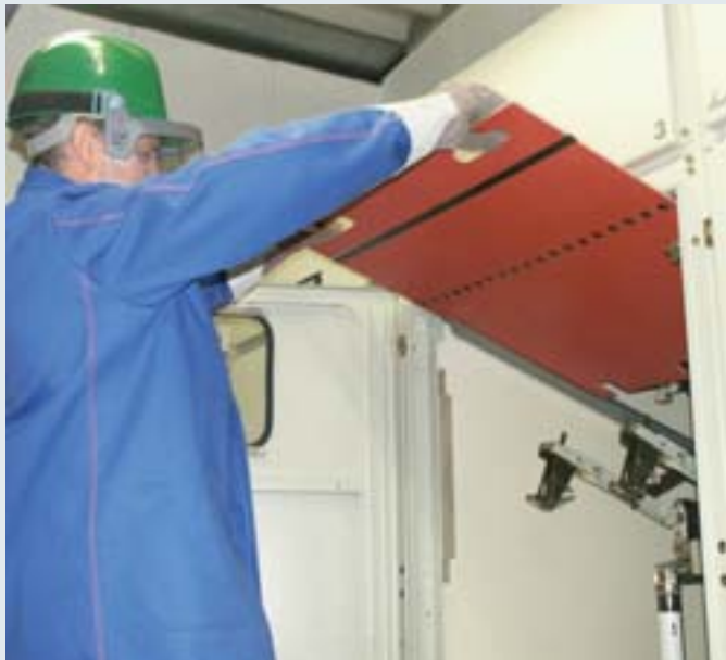
Inserting a protective shutter, type A1 by hand
