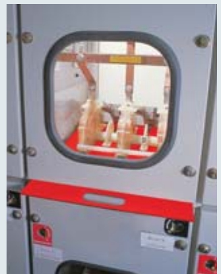
Inserting an insulating protective shutter, Type A4.
