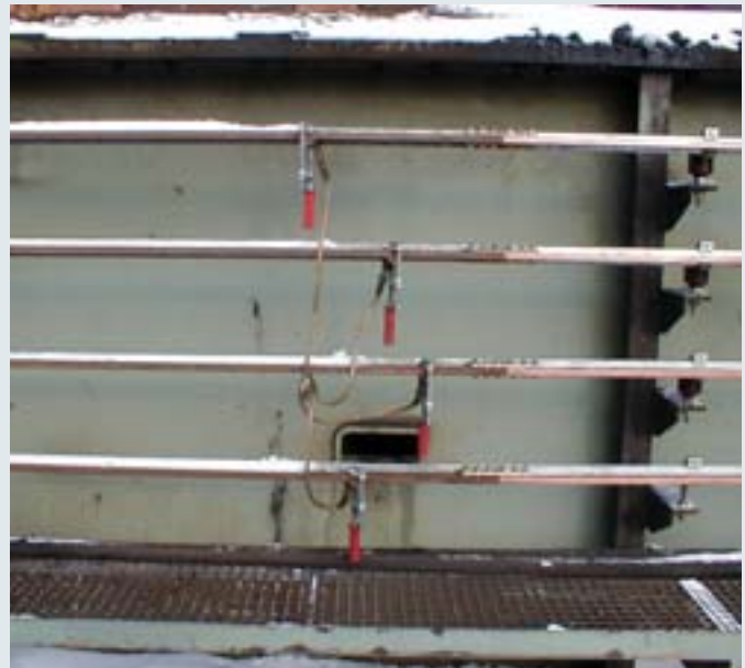
Four-pole earthing and short-circuiting device with clamps.
