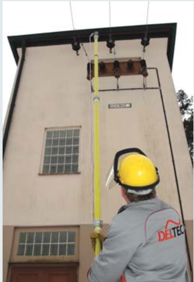
Earthing rod consisting of a top section, intermediate section and base section.
