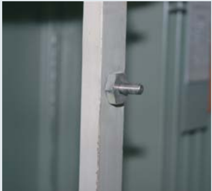
Earth connector with threaded M12 pin for bolting to an earthed part of the installation.
