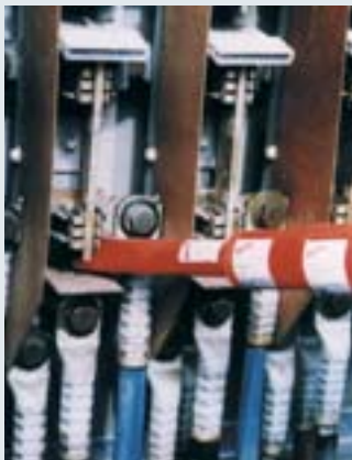
Chamfered flat cleaning head in use.
