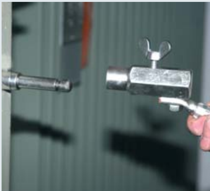
Fixed earthing point with grooved ring and earth connector.
