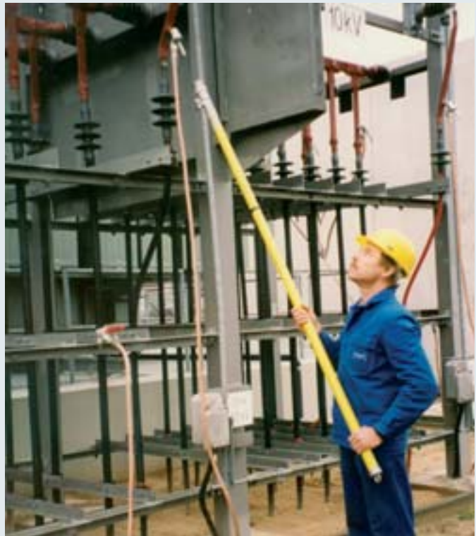
Rigid ball head cap with long shaft and earthing rod.
